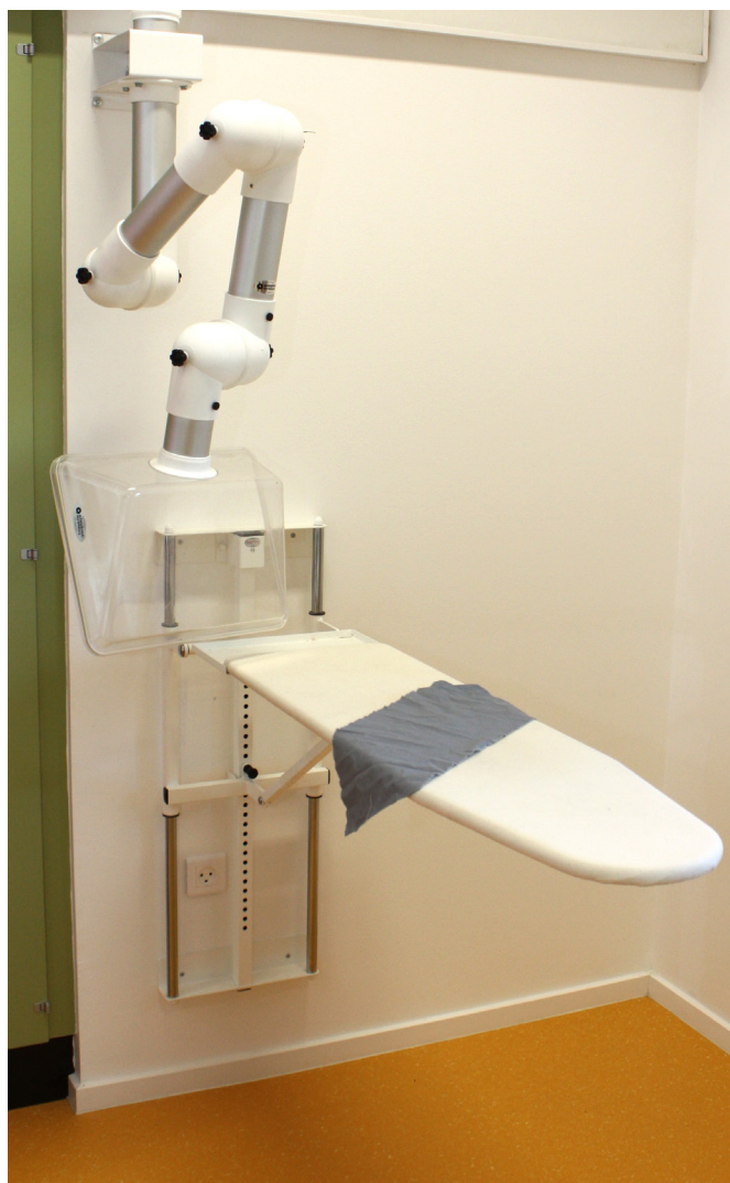
Height adjustable ironing board with compulsory point exhaust
