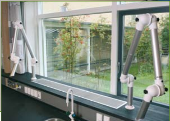
▲ Pupil workstations along the wall containing installation casing for water, electricity, gas, and IT. Note the covering grating for the radiator.
