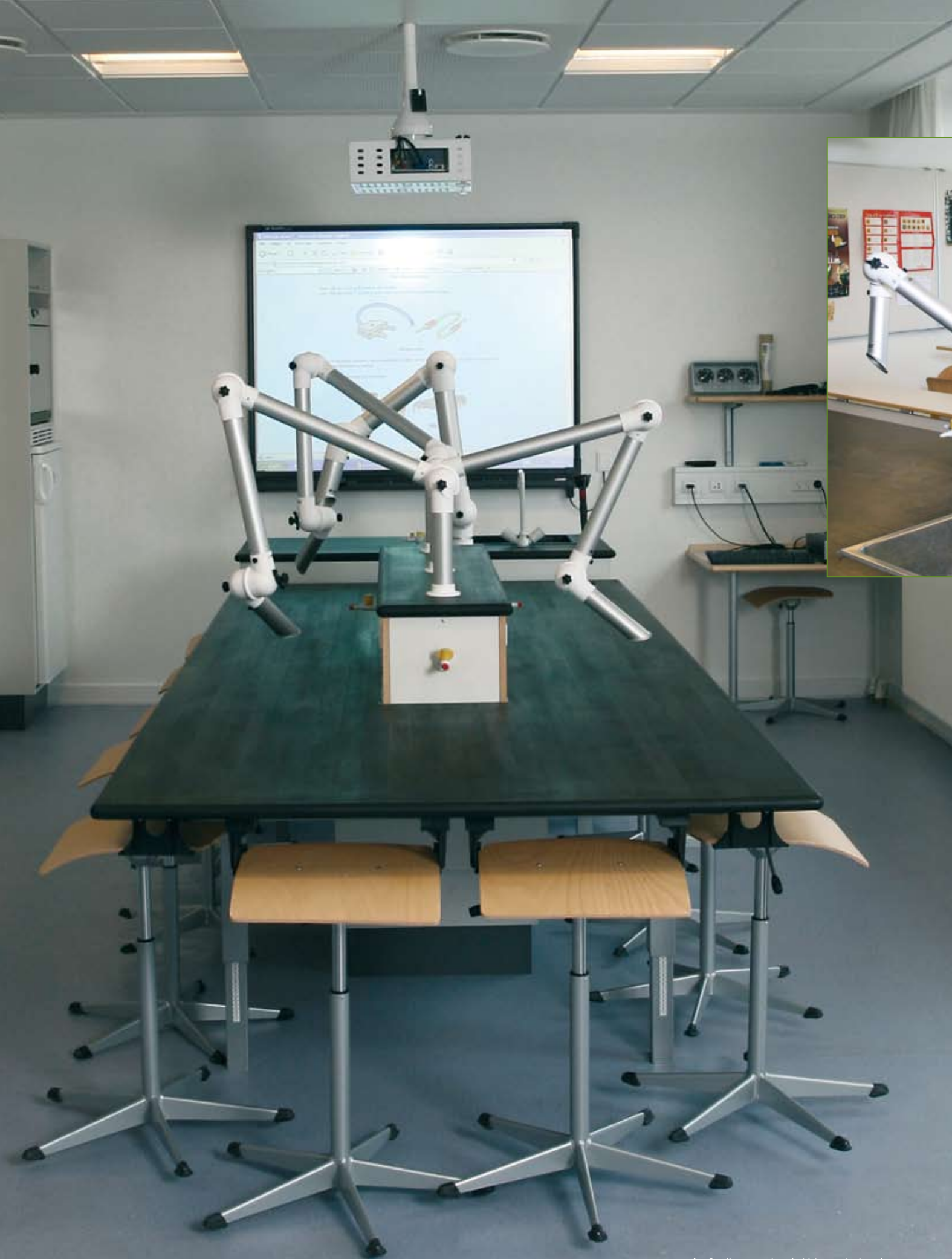
▲ Small room equipped with interactive board. Note the hanging stools and local extraction in the panel box.
