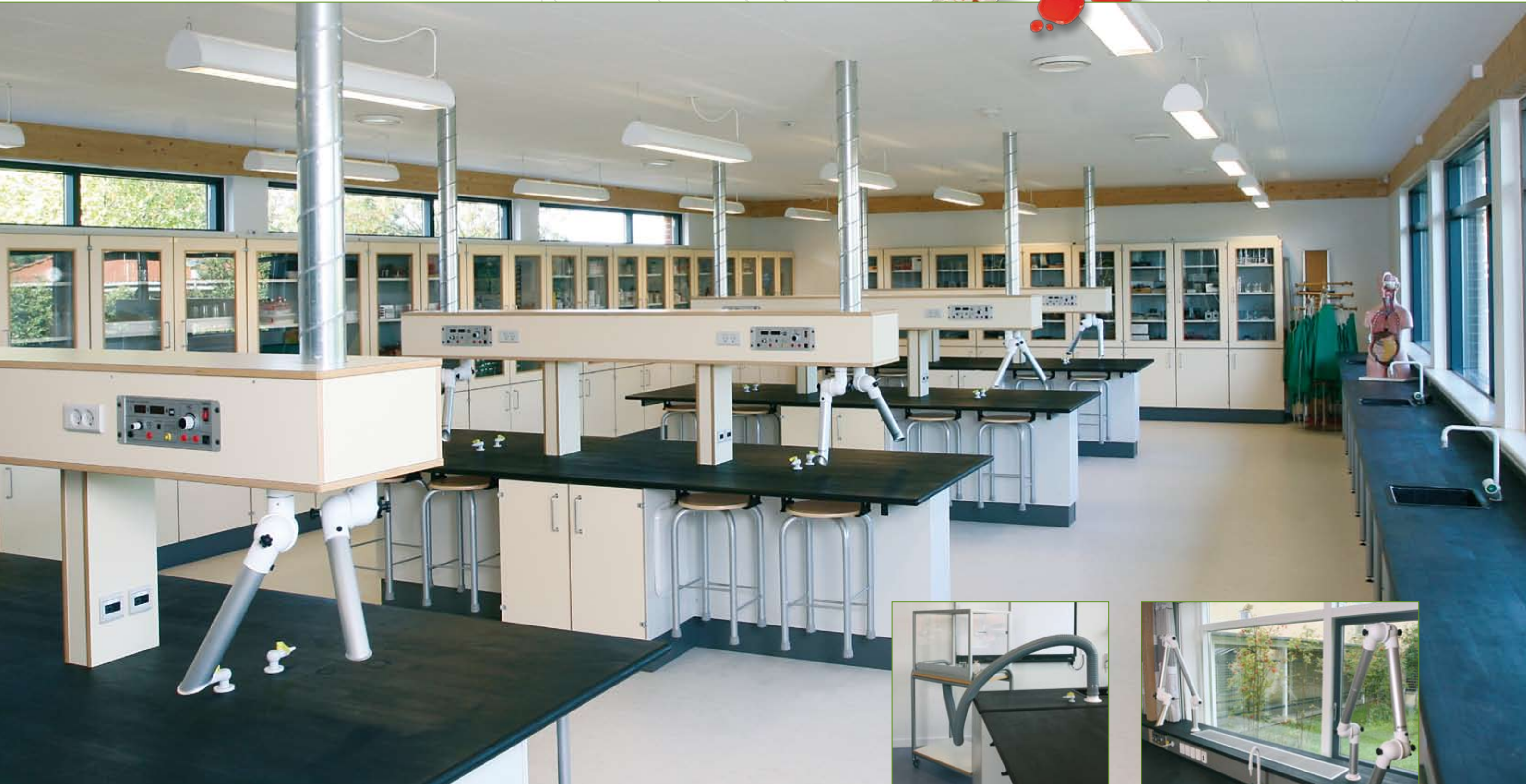
▲ Mobile extraction hoods facilitate flexible demonstration.
